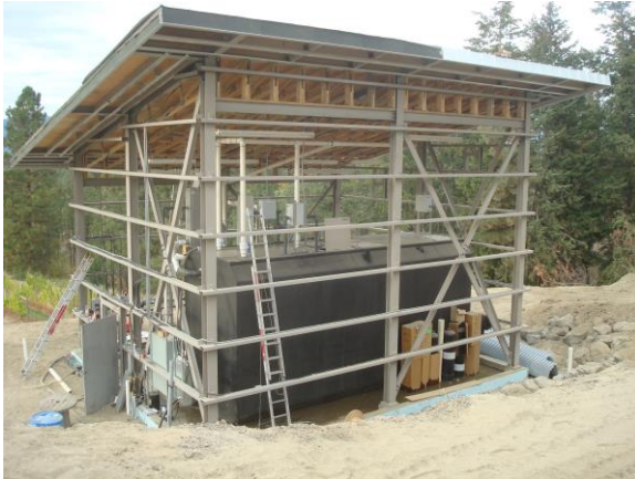
Under construction with building
