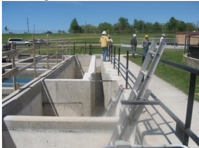
UV Channel Under Construction
