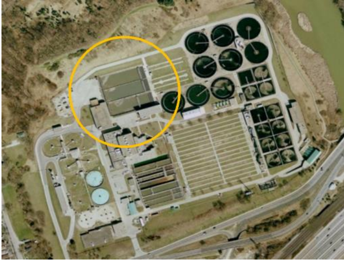
Humber WWTP Clarifiers
