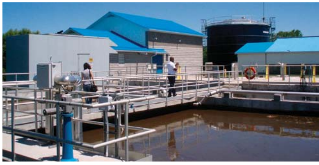
Norwood Water Pollution Control Plant.
